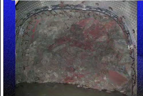
SHOTCRETE ARCH, 2M SPACING, SPAN 6.8m, 6" SHOTCRETE, SPILING UNDERNEATH ARCHES
