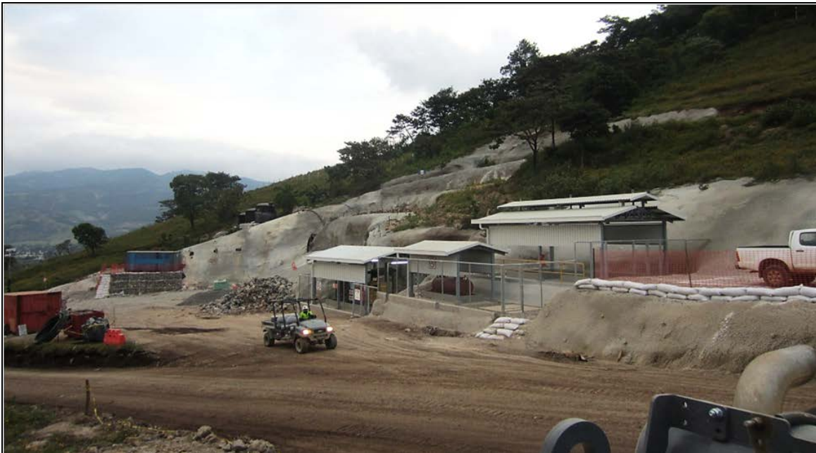
Figure 16-2: West Central Decline Portal Area
